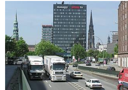
66,8 mill. m 2 street infrastructure
